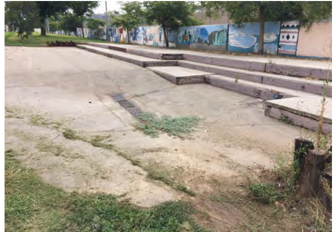
Old and unused concrete foundations, surrounded by dirt and dead grass
