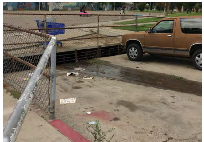
Large storm drain located at the end of Vanegas Lane
