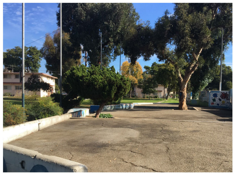
Old concrete and asphalt
