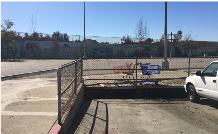
Catch basin drains runoff into storm drain under project site
